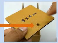
• Lay the housing flat with the open side facing up. Measure 9 cm from the bottom.
